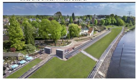
The Dutch Float Dike (DFD) is a self-activating flood barrier that uses the force of incoming water to provide reliable protection. The concept is simple yet powerful: as water rises, the barrier floats up into position, automatically securing the area against flooding. When the water recedes, the system drains and the barrier resets itself—ready for the next event.
